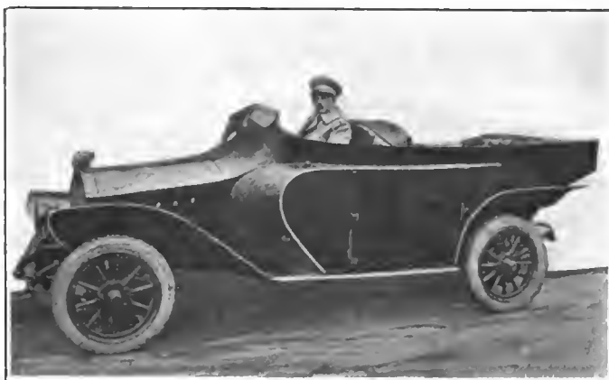
Side view of the all-enclosing carriage body placed upon a Benz chassis by the Delmenhorst Wagon Company
